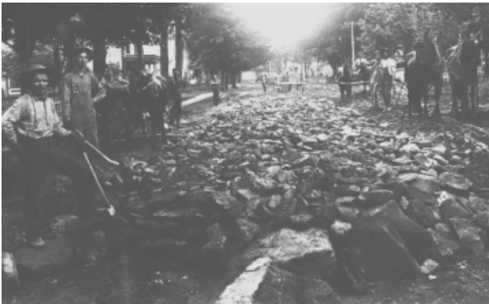
Below: Putting in a stone base on Main St.
