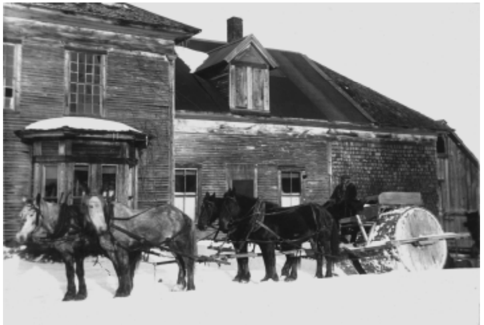
Howard Carpenter rolling the roads.
