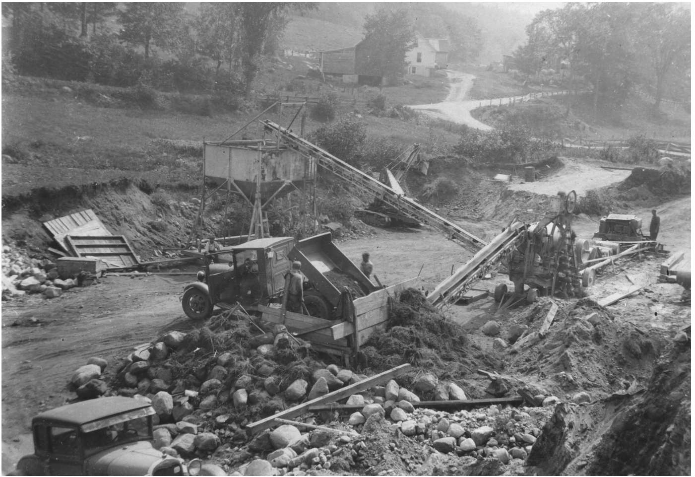
Above: Sifting out the stones at the gravel-pit, circa 1930. The house in the background is the present home of Charlie Pilbin.
